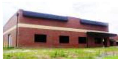
MoldStoppers is moving into this building in the Southern Pines Corporate Park.
